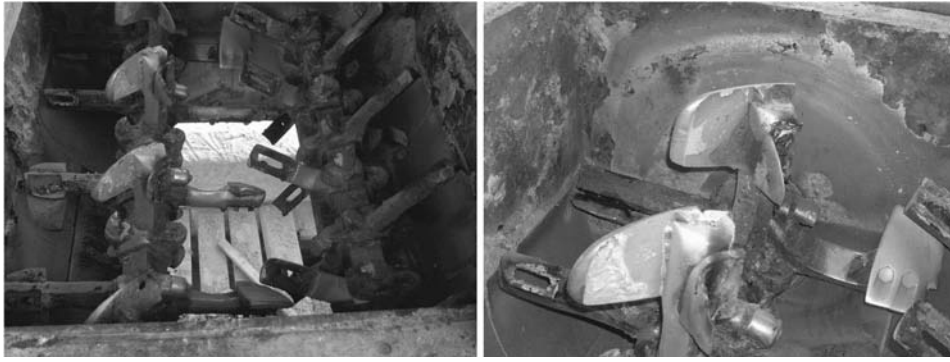
Figure 9. Interior view of blades installed in asphalt mixer
